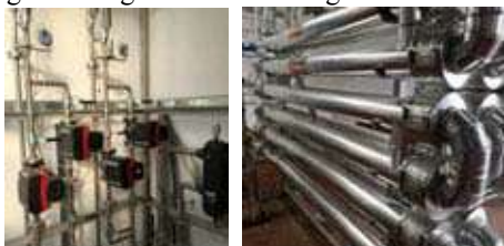
Fig. 4. Circulation pumps and secondary sludge-water HEX.
