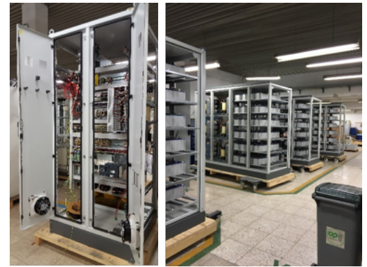
Fig. 4. TF power supply charger (left) and part of the TF ultracapacitor banks (right).
