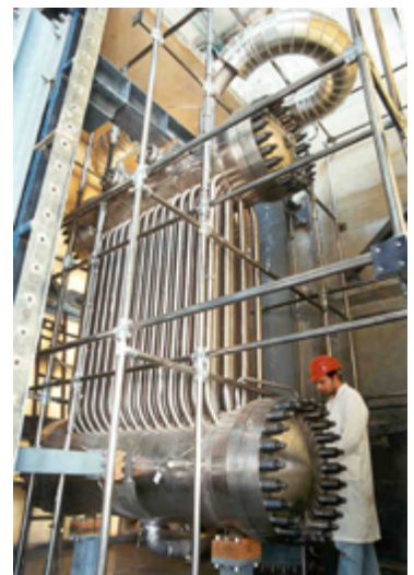
SBWR Isolation Condenser testing on the PANTHERS facility (power: 20 MW)
