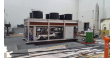
Dynamic/functional test on air treatment components
