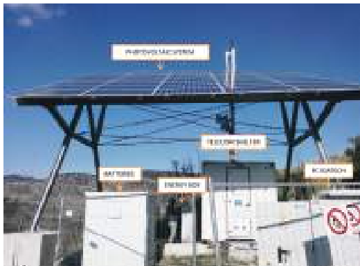
Fig. 2. FC-powered RBS site installation: site#1
