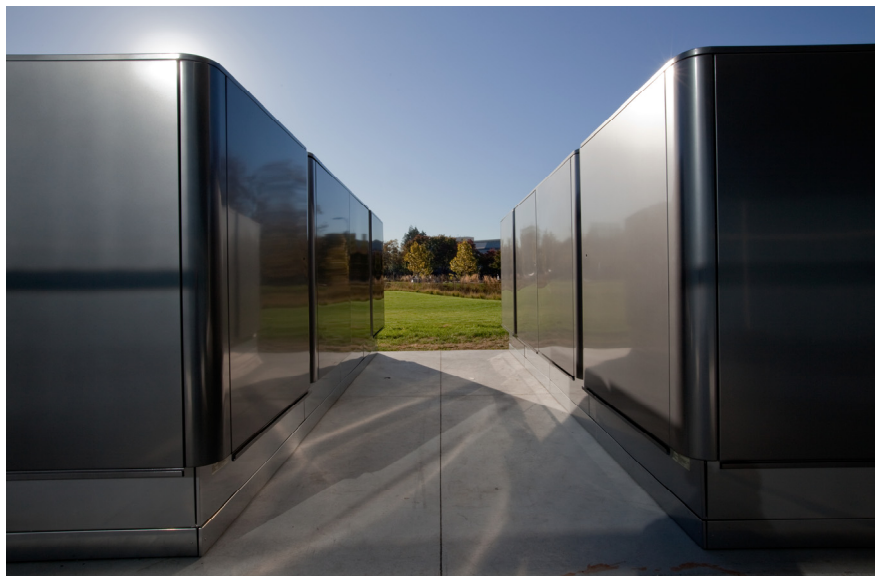
FIGURE 156 Apple 10 MW SOFC farm made up of 50 Bloom Energy boxes rated 200kW each in Conover, North Carolina 4
