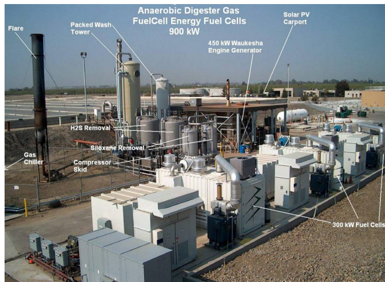
FIGURE 27 Original installation of Three FuelCell Energy Fuel Cells and Gas Pretreatment Unit at Tulare Wastewater Treatment Plant
