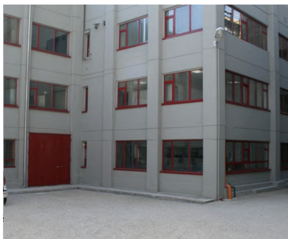
Fig 2 South-west wing of the building: first and second floor are occupied by MW labs
