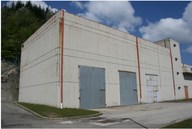
Fig 3 View of exPEC “CHILLED WATER BUILDING”
